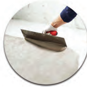
Comprehensive Floor Prep
