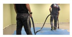
5. Pump Schönox self-leveling compound to desired thickness.
